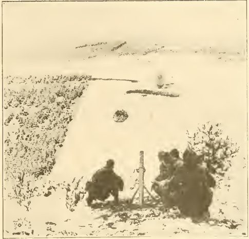
DEMONSTRATION OF BRACKET FIRE
