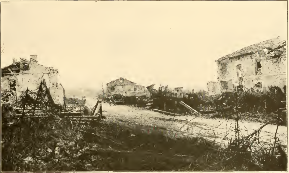
THE HIGHWAY INTO FRESNES-EN-WOEVRE
