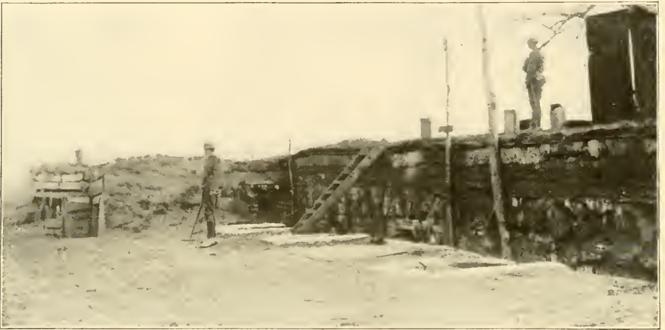
CONCRETE WALLS FIVE FEET THICK
