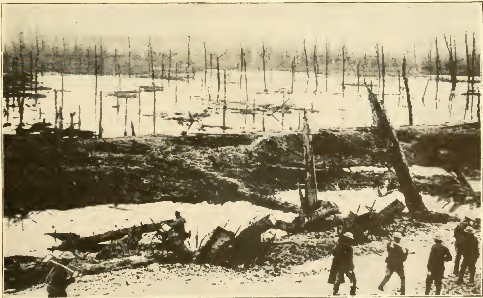
ON THE ANCRE RIVER, WHERE THE BRITISH ADVANCED IN MIDSUMMER OF 1918
