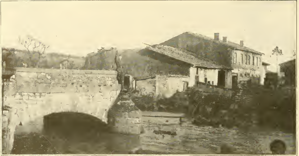
THE BRIDGE AT PAROIS
