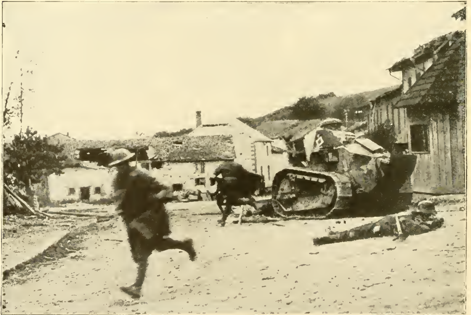
A DANGEROUS CORNER IN EXERMONT
