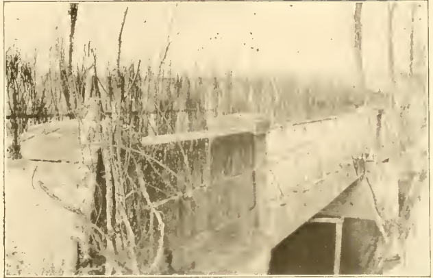
THE APPROACH TO CONSENSVOYE BRIDGE
