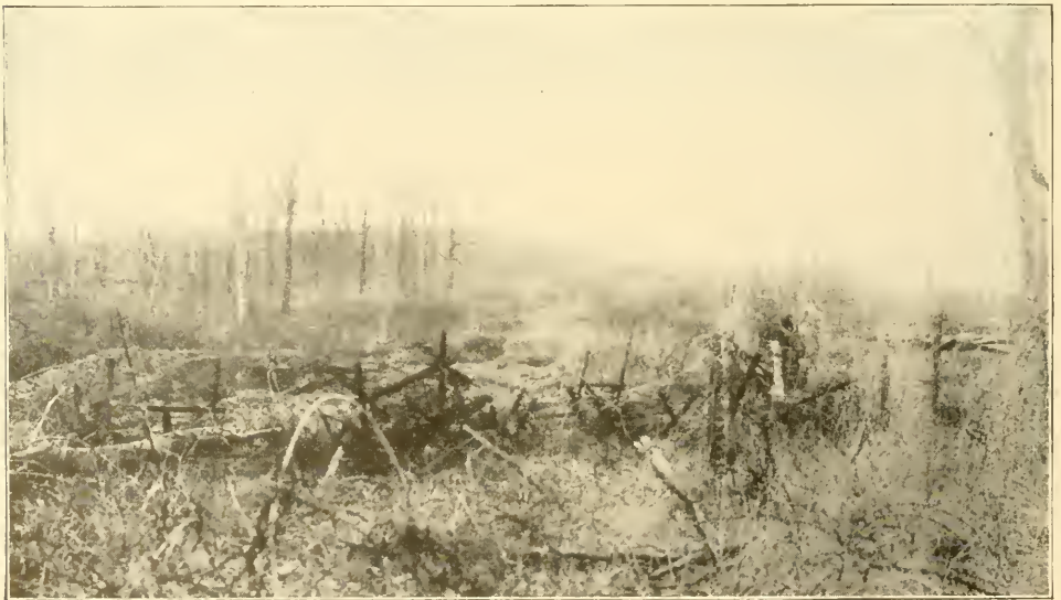
ON THE SLOPE OF LA CIGALERIE
