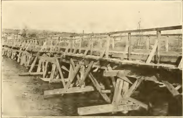
THE WORK OF THE 108TH ENGINEERS One of the bridges over the Meuse at Consenvoye.
