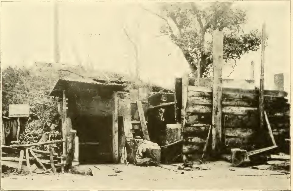
GERMAN ELECTRIC POWER PLANT AT GERCOURT
