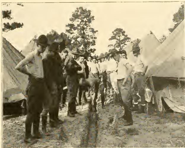
AND SOME DUG DITCHES
