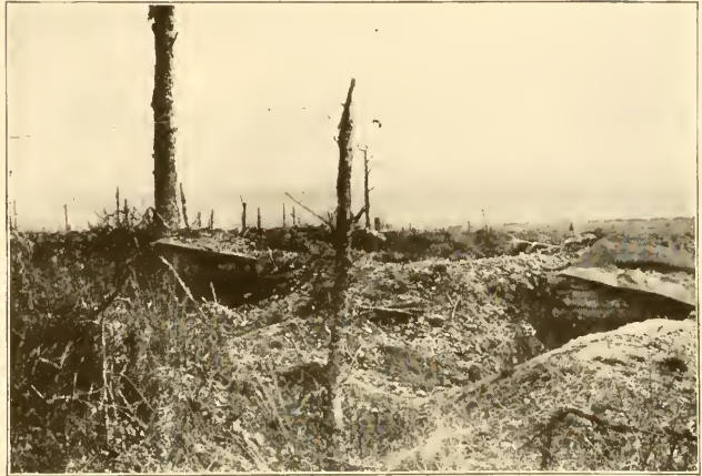
GERMAN OBSERVATION POST IN CERVAUX TRENCH
