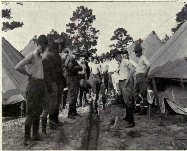
AND SOME DUG DITCHES
