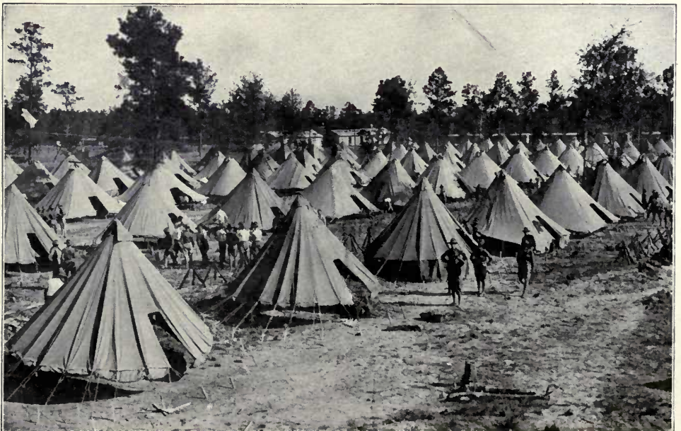
GENERAL VIEW OF THE 132ND'S CAMP
