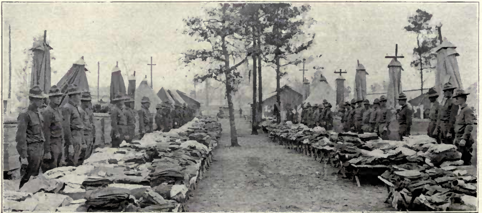
INSPECTION AT CAMP LOGAN
