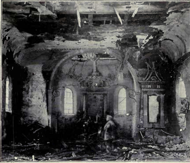
INTERIOR OF THE CHURCH AT DANNEVOUX
