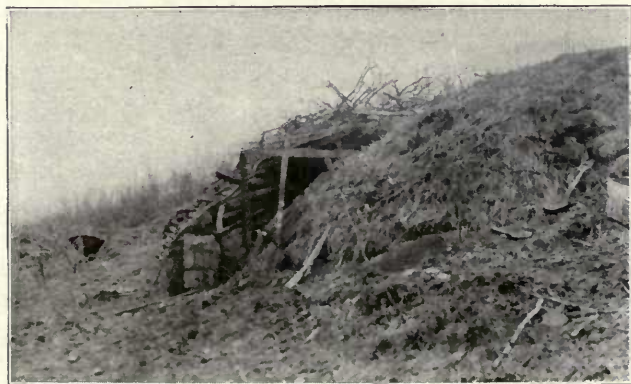
ADVANCED HEADQUARTERS OF MAJOR ALLEN IN DEATH VALLEY SOUTH OF THE BOIS DE CHAUME
