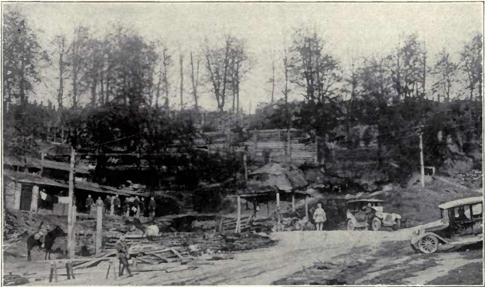
GENERAL VIEW OF BRIGADE HEADQUARTERS
