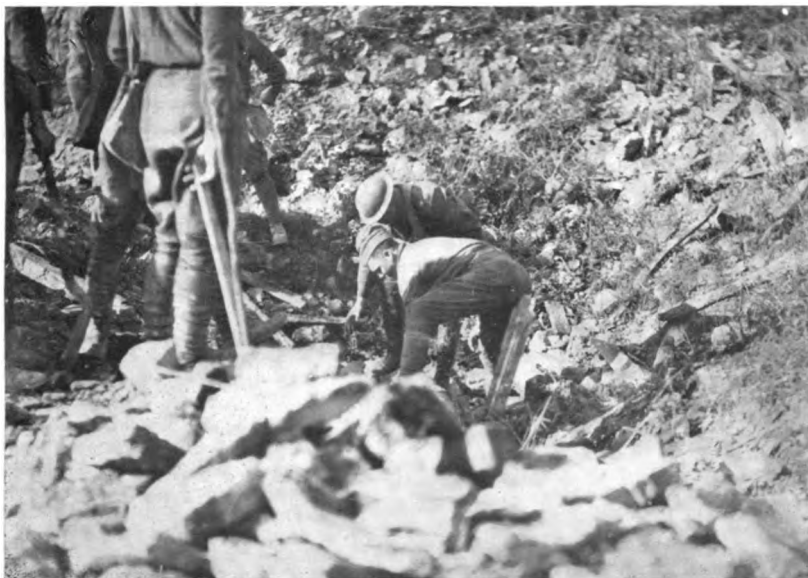
ERECTION OF REVETMENT WALL OVER SHELL HOLE, FORGES ROAD
