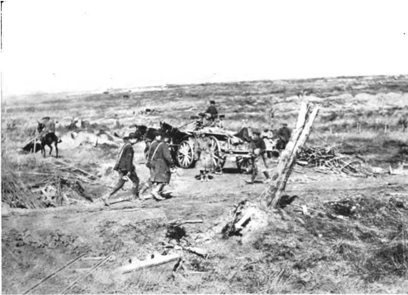
BEGINNING OF NEW CUMIÈRES-RAFFECOURT ROAD
