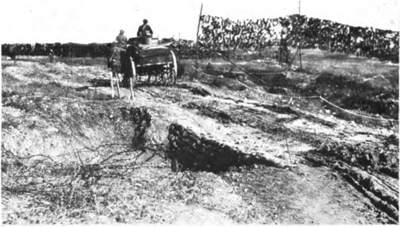
CUMIÈRES-RAFFECOURT ROAD, CUMONT RAVINE
