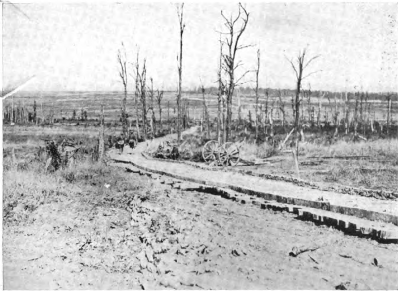
CORDUROY ROAD, SOUTH END OF FORGES CREEK SWAMP
