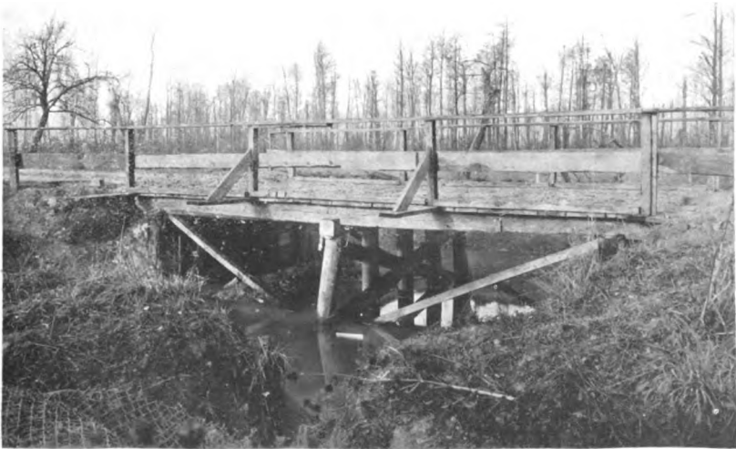
BRIDGE ON HARVILLE-MANHEULLES ROAD, TROYON SECTOR
