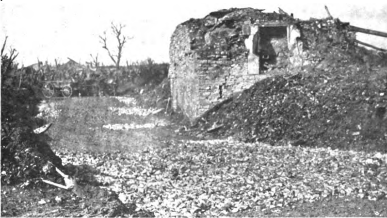
COMPLETED SECTION OF FORGES-BÉTHINCOURT ROAD
