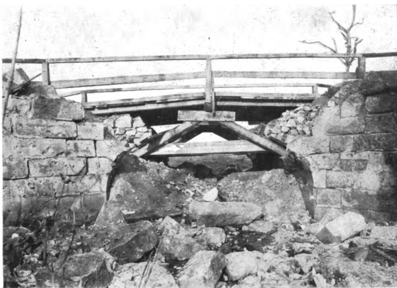
BRIDGE ON HARVILLE-MANHEULLES ROAD, FORGES SECTOR
