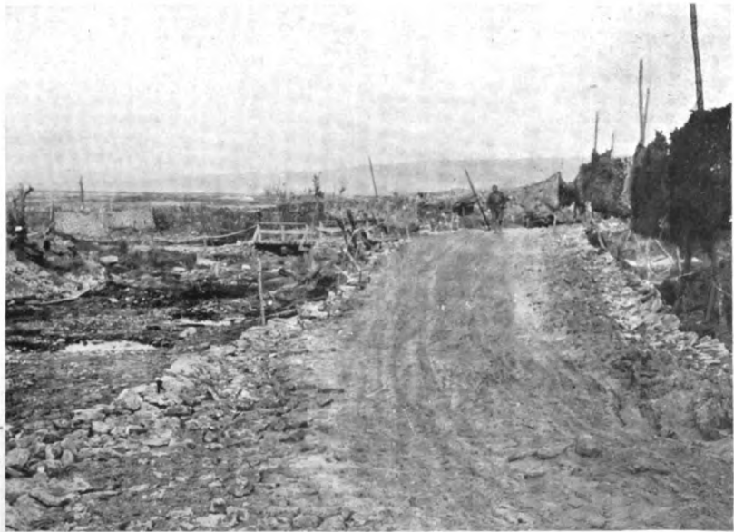
ROAD OVER FORGES CREEK BRIDGE
