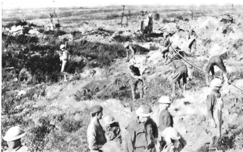
CONSTRUCTION OF FORGES-CONSEVOYE ROAD
