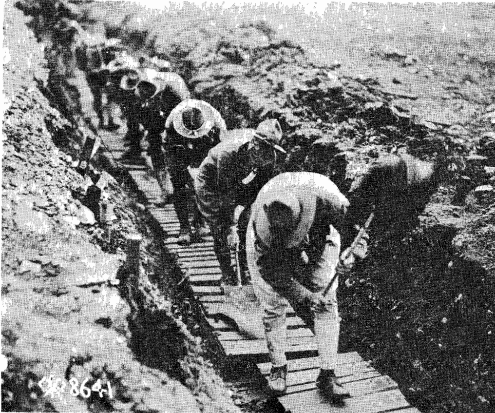
Recruits at Camp Kearney, California, using British Ayrton or trench fans to clear gas, 1918.
